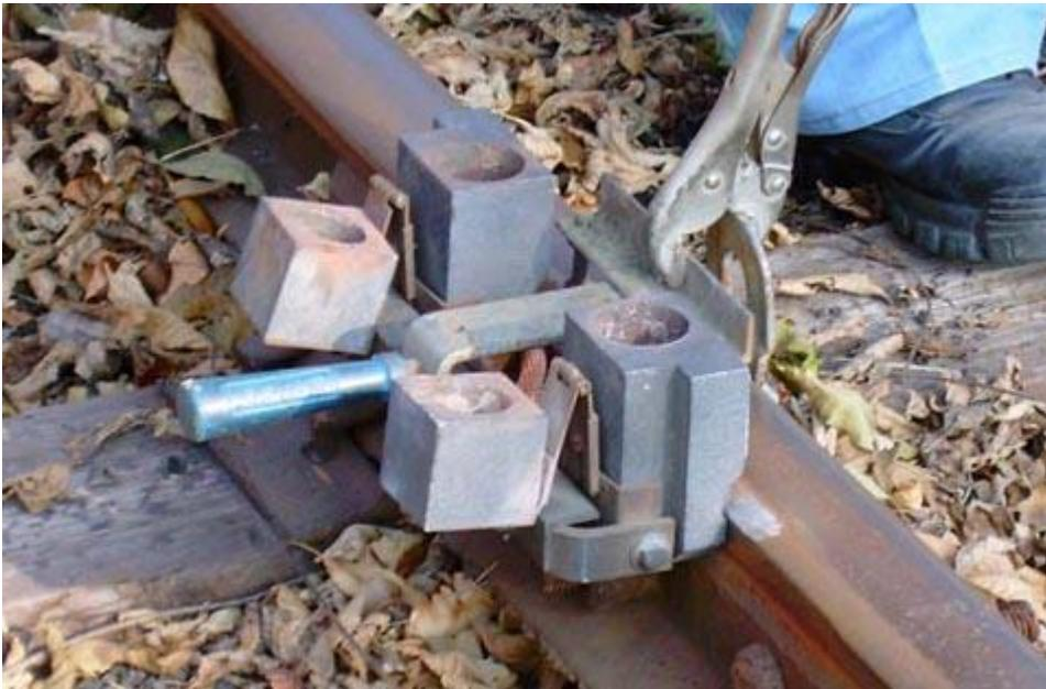
**After the rail heads are prepared, the mold is attached. The mold has cavities to hold the ignition charge and weld material.**
