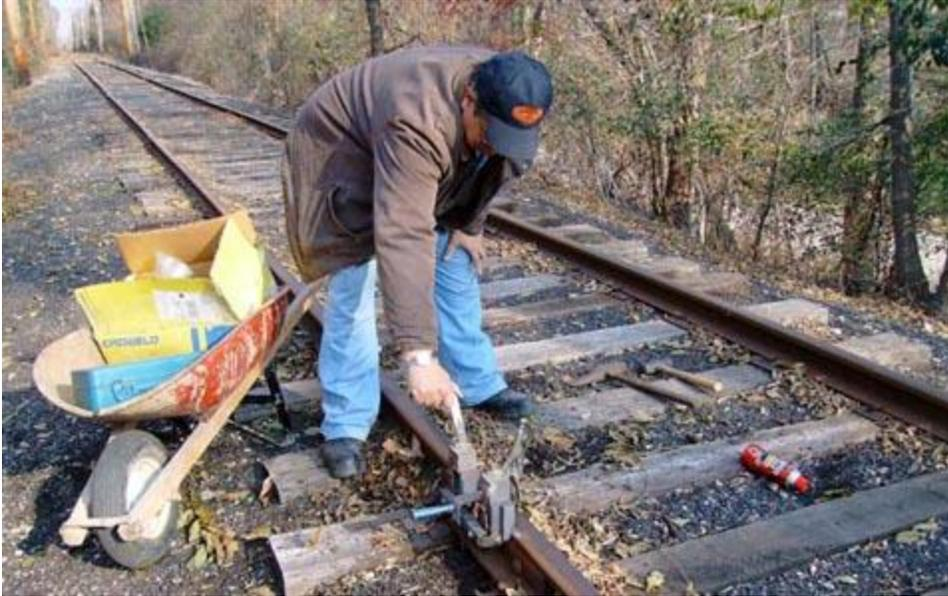
**When the mold is attached, the cavities are filled with both a thermit charge and an ignition charge. The ignition charge is ignited by sparks from a special "lighter."**
