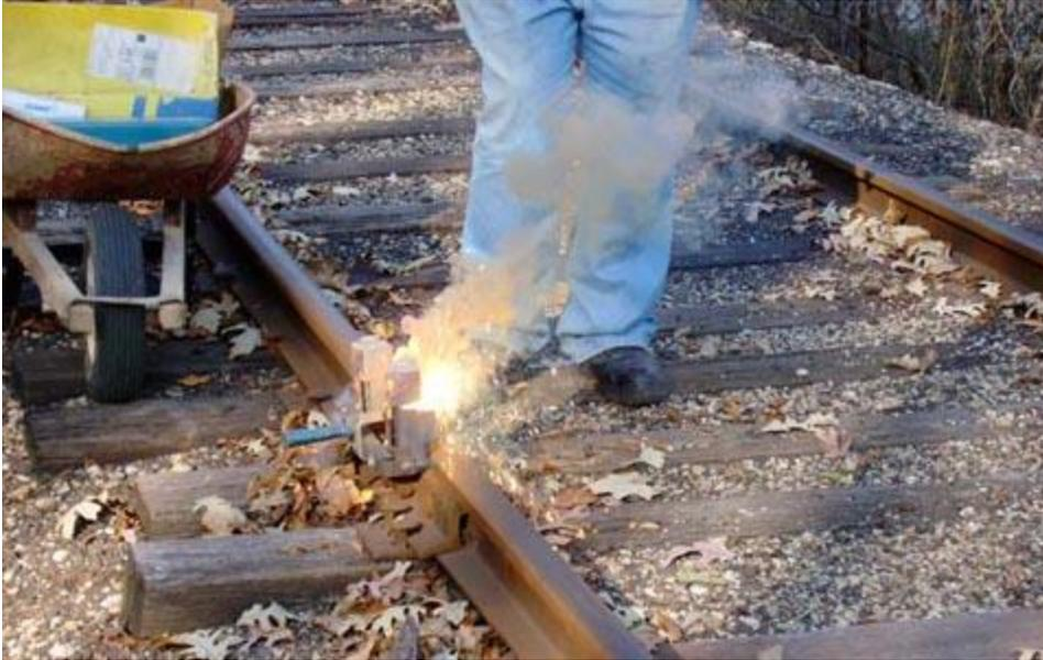
**The weld takes place after ignition. The charge heats the welding material to 4000 deg. fahrenheit. After cooling the mold is removed and cleaned of residue and made ready for the next weld.**
