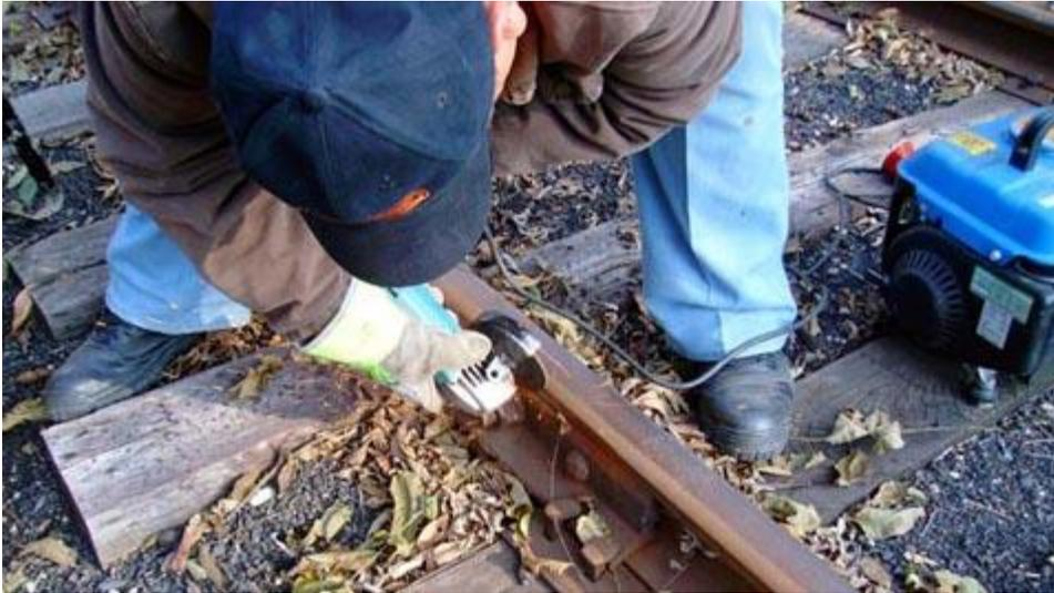
**The rail heads at the joint must be prepared to take the weld. This is done with a powered grinding wheel or steel brush. A steel brush is used here.**
