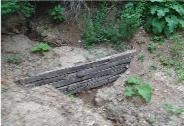
**Last season saw the completion of a retaining wall at the culvert near Stop 52. This has stemmed the flow of water and clay over our tracks.**
