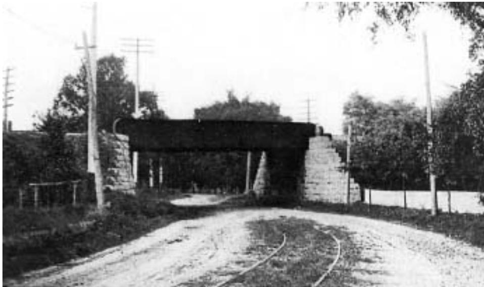
**The second crossing at grade with the C&NW was avoided as seen here. Going north under the steam road the track made an abrupt turn to the west and headed toward Third Street in Geneva.**
