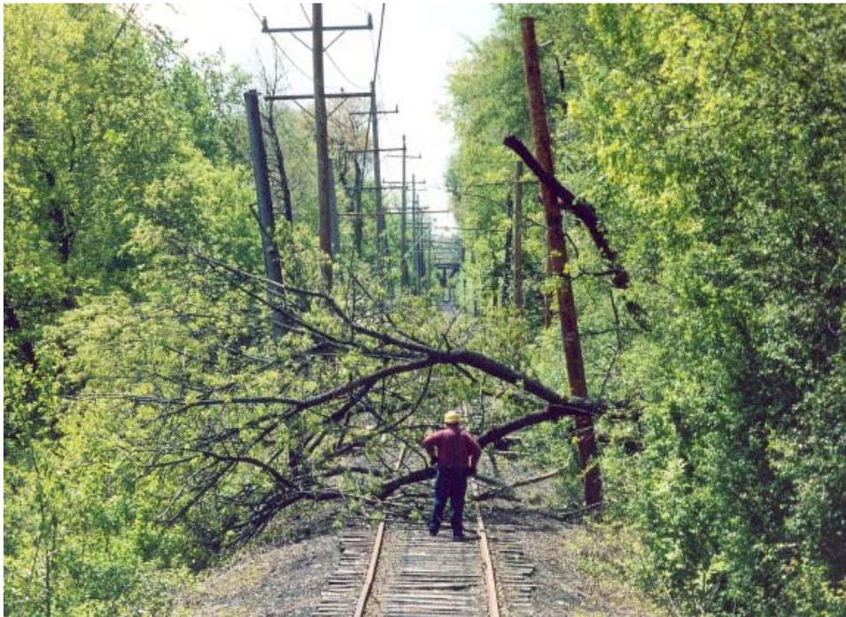
**Fred Lonnes surveys fallen tree and damage to trolley wire and feeder line at pole 22. Monday, May 12, 2003.**
