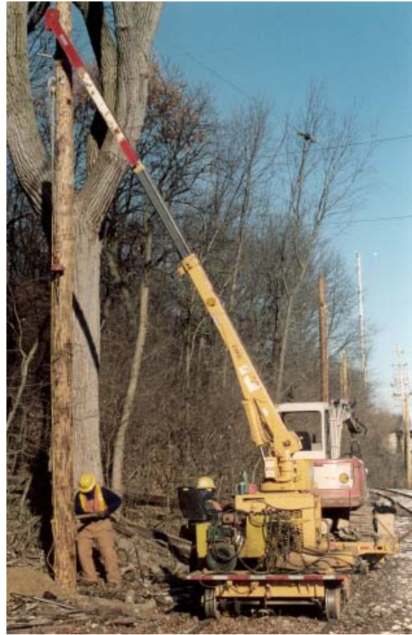
Left: Attaching "trolley wire" to a "span wire."
