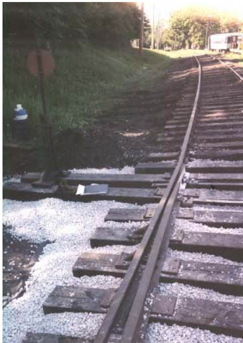
The CRANDIC switch point being installed in the mainline - April 2001.
