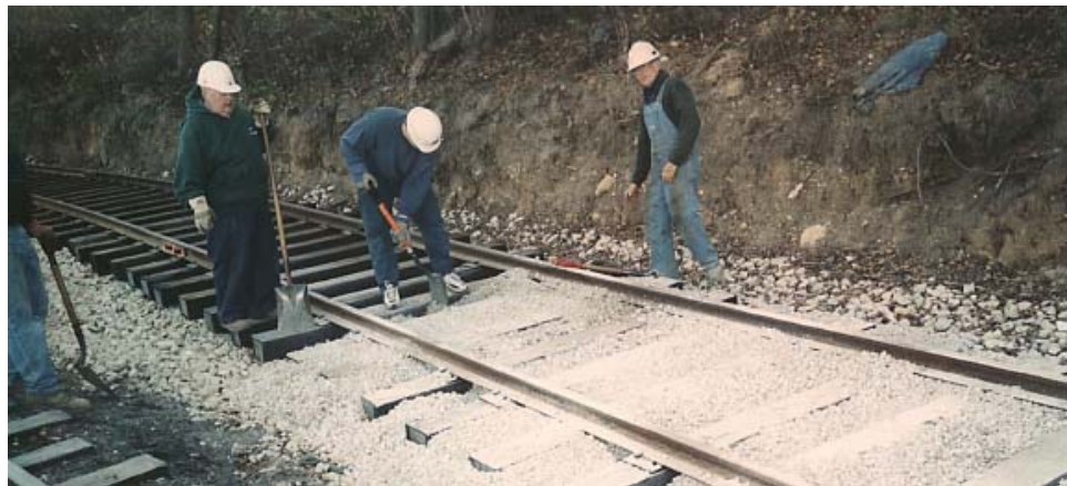
Ballasting and surfacing on Track One West - October 2001.
