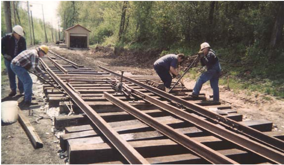
The frog from the CRANDIC is in place - April 2001.
