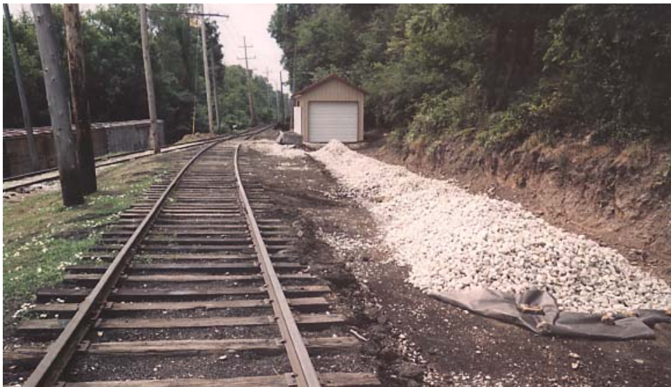
The fresh stone in place ready for ties - July 2001.
