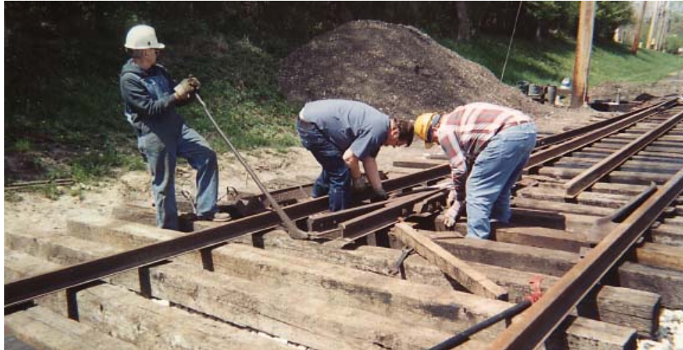
Placing the "frog" for the MOW switch. A real heavyweight job.
