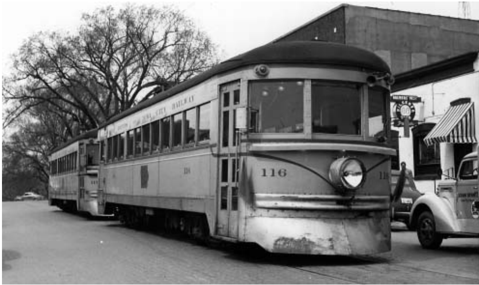
CR&IC 116 AND 117 on Saturday, April 10, 1948 preparing to the leave the Iowa City station for Cedar Rapids. Note the flags (green) on 116. The Ex C&LE cars did not have drawbars so when traffic demanded trains were run in sections.
