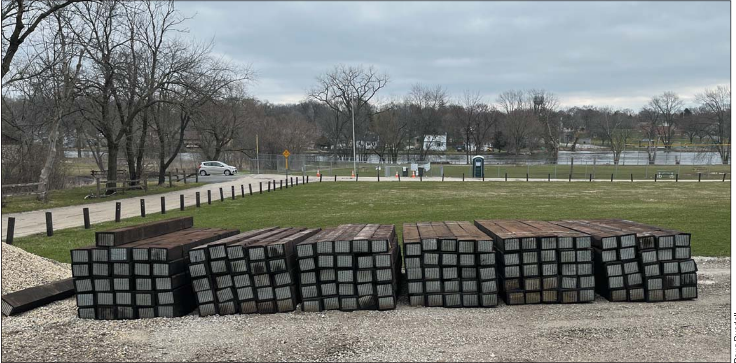
Some of the new tie bundles in the parking lot before installation started.
