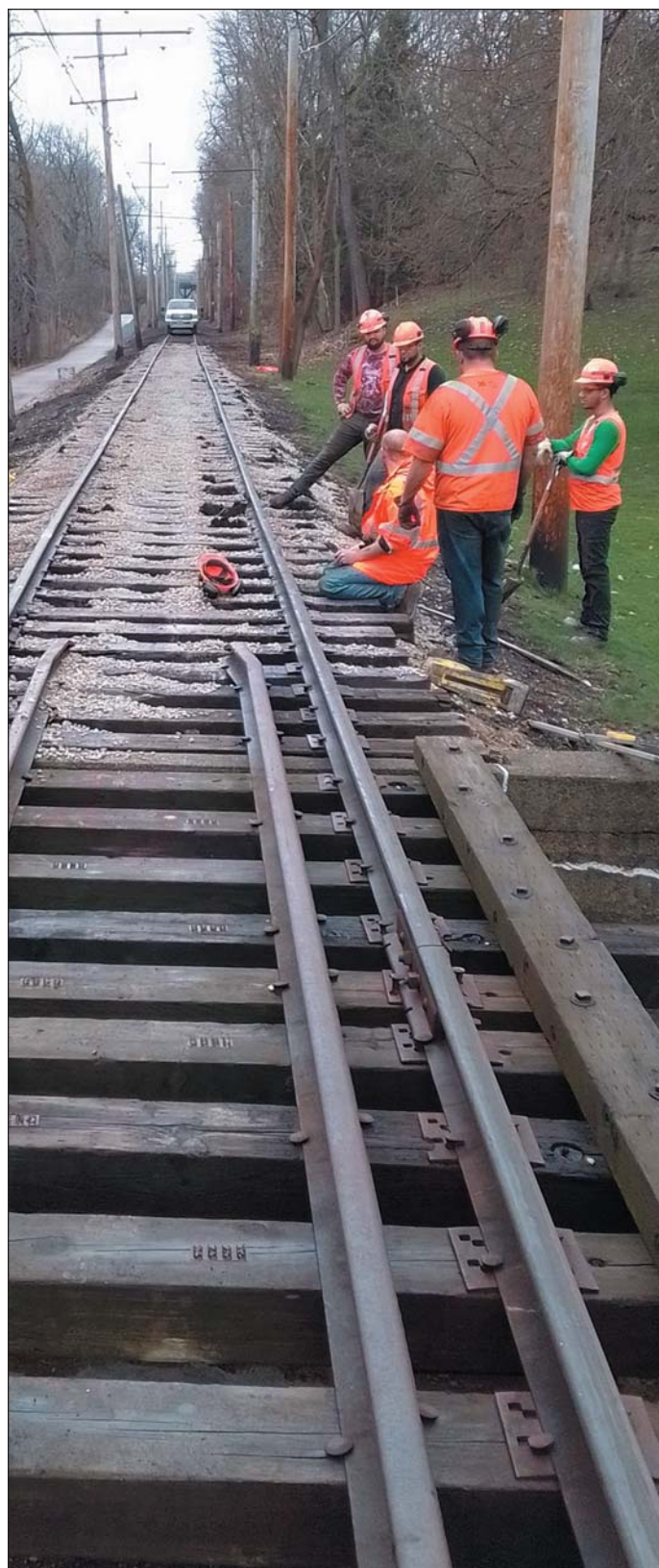
Surfacing the track so both rails are even so our cars have a level ride.
